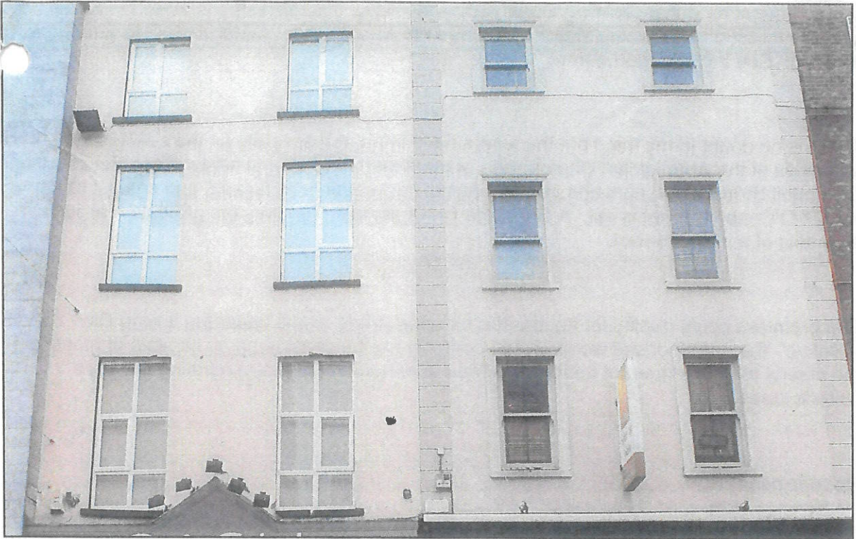
Plate 3: View of the upper floors of 27 and 28 O'Connell Street, the latter having retained rise-and-fall sash windows, as recorded on February 8, 2017.
